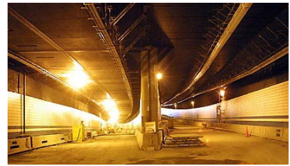
2002 Central Artery Tunnel "The Big Dig" Boston, MA, USA
