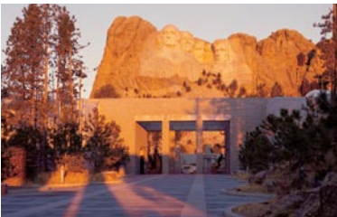
1997 Mount Rushmore National Memorial Visitor Center Blackhills, SD, USA Plaza and Deck Installation over auditorium
