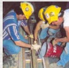
Epoxy resin grout cures at normal temperatures into a tough, non-shrinking, structural grout of high chemical resistance. L&M EpogROUT 758™ is scientifically formulated to withstand severe dynamic load shock in marine and heavy-duty industrial applications.
