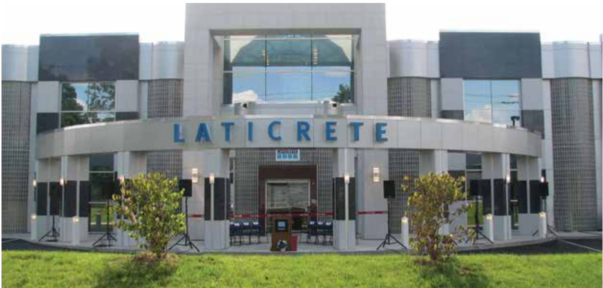
LATICRETE International, Inc., Headquarters, Bethany, CT
